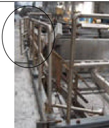
Pot Line – The handrail in place will protect the stage till the new pot setting.
